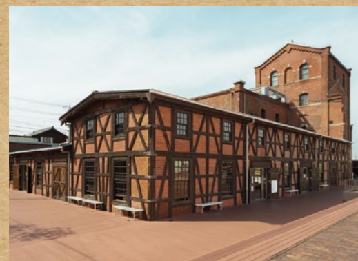
Handa Red Brick Building — Aichi
